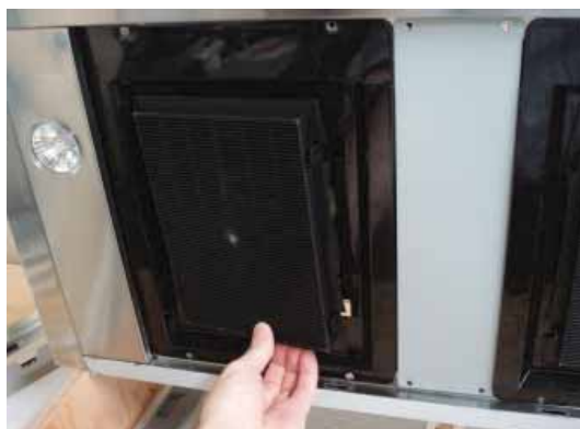
3. Install charcoal filters into charcoal filter brackets
