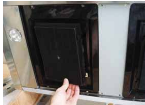
3. Install charcoal filters into charcoal filter brackets
